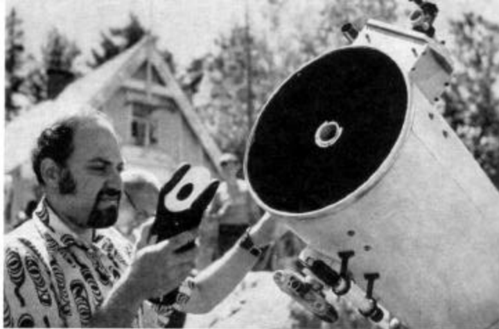
Above: Albert Nagler with the perforated diagonal of his 12-inch reflector, which is described in the text.
